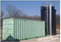
Figure 2: A dosing station (22 m<sup>3</sup>) and a container with a mixing tank inside.
